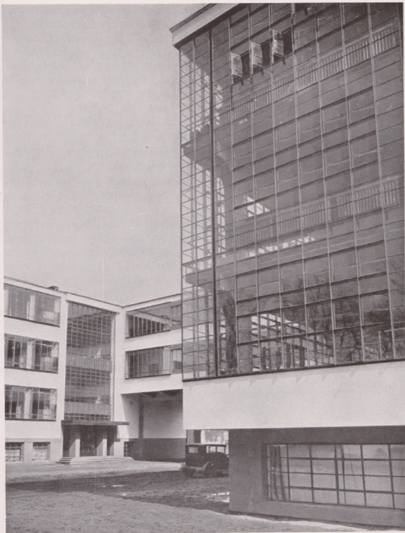
230. WALTER GROPIUS, The Bauhaus, Dessau, 1926. Corner of the workshop wing. In this case it is the interior and the exterior of a building which are presented simultaneously. The extensive transparent areas, by dematerializing the corners, permit the hovering relations of planes and the kind of "overlapping" which appears in contemporary painting.
