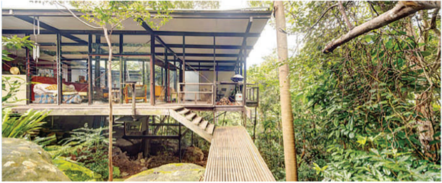
12. The Lucas House entry elevation. The approach is through the bush along a suspended wooden walkway that has no handrails to emphasise its openness, Caroline Simpson Library, Museums of History NSW Collections, Ray Joyce
