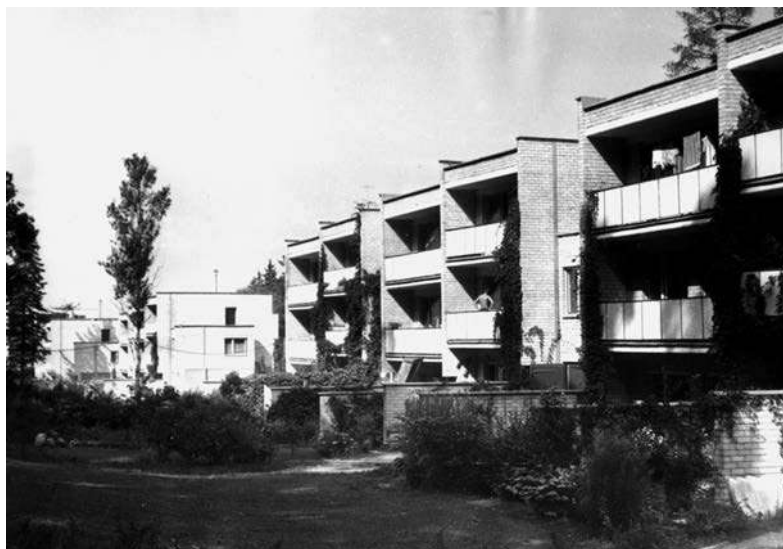
12, 13. Artists' housing cooperative in Vilnius. Post-construction photos. 1975
