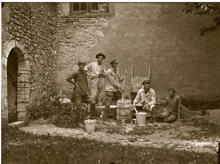
3. Professor Helge Kjellin and his team of conservators during the renovation of the 13th-century Ridala church in western Estonia. From left: Kjellin himself, construction surveyor and student at Tallinn College of Engineering Nikolai Paulsen, art history student Georges Liedemann, student at Tallinn Industrial Art School Heinrich Hein, and art history student Helmi Saarmann (Saadre at the time). 1924
